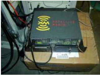
XM repeater at Mt. Harvard near Los Angeles - photo courtesy Frank Martin
